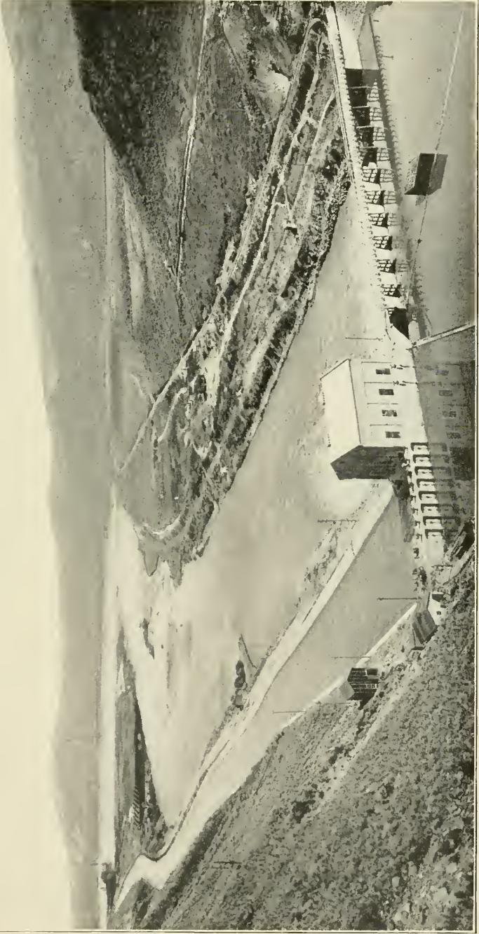
VIEW OF THE BOISE HYDRO-ELECTRIC POWER PLANT AT BOISE, IDAHO The plant develops 2000 horsepower which is transmitted about twelve miles up the River to Arrowrock Dam site where it is used for construction purposes
